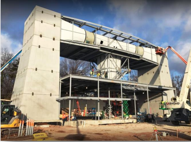
Model 14R4 Under Construction
